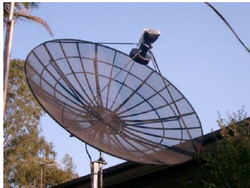
Fig.2 3.7 metre diameter parabolic dish for 1296 and 2301 MHz EME operation SCARC member Wayne VK4WS set up the feed horn for VK4AFL.
